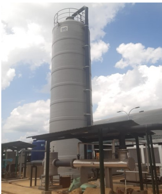
Image: Biogasclean biogas scrubbing column (Source–Biogasclean).
