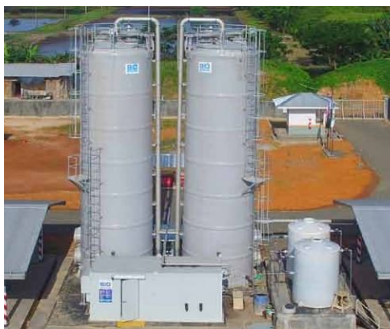
Image: Biogas column scrubber (Source–biogasclean.com).
