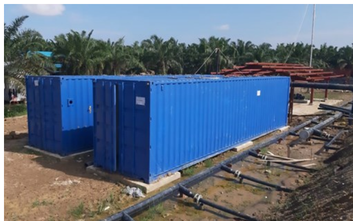
Image: Elmoz biogas biological scrubber installed at PT. Pasadena Biofuel Mandiri (Source–PT. Elmoz GEO Solusi).
