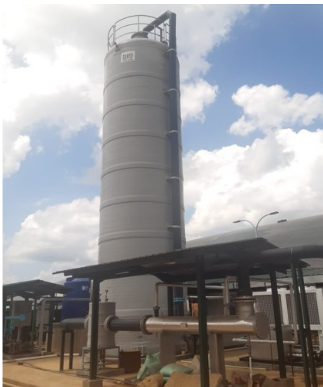
Image: Biogasclean biogas scrubbing column (Source–Biogasclean).
