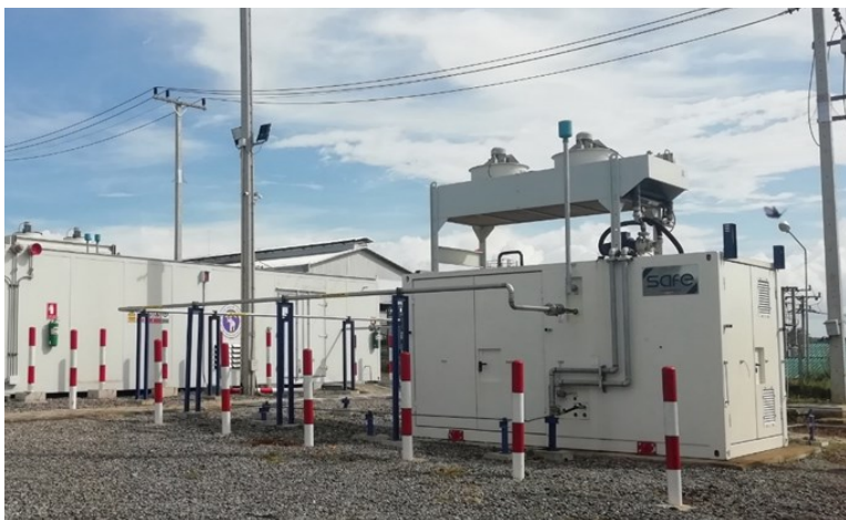
Image: Biogas upgrading and compression skid system (Source–Safe S.p.A.).
